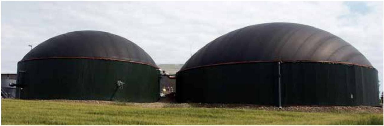
*Figure 5.5 Anaerobic Digestion can be used to convert slurry into organic fertiliser, while the waste gas can be collected and used as a fuel. Picture from Irish Independent*
