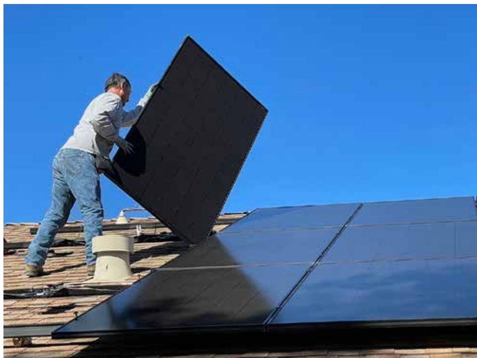
*Figure 5.1 Installing 12m<sup>2</sup> of rooftop solar PV panels can provide about 25% of the electricity needs of a typical Irish family. Photo by Aldo De La Paz on Unsplash.com*
